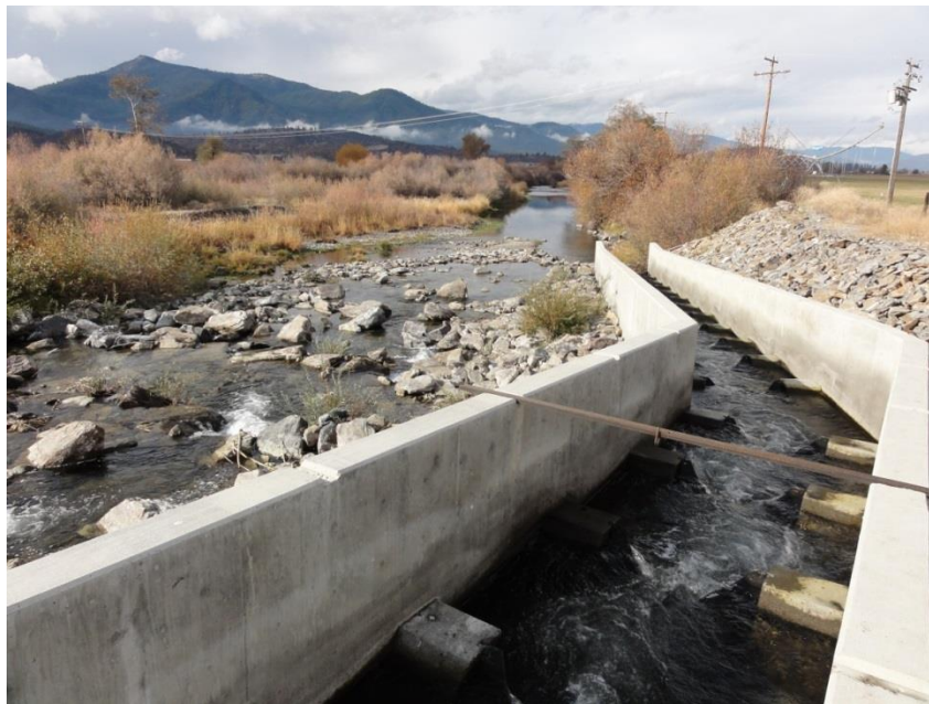
Figure 28. Scott River at Young's Dam and fish ladder on 11/13, end of lease.
